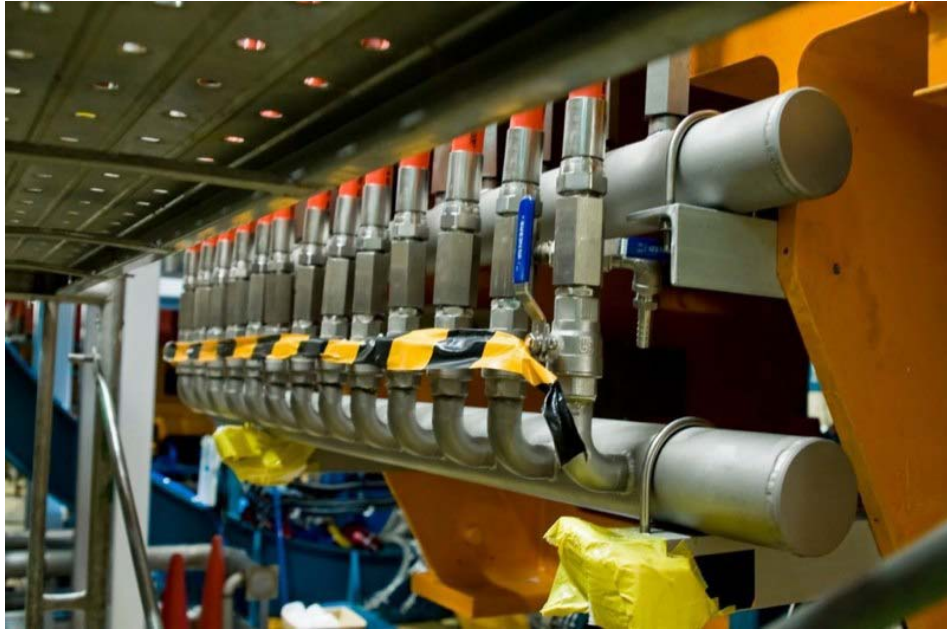
Fig. 4. The magnet water manifolds during installation in August 2009.
