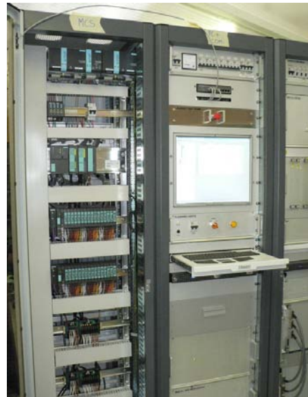
Fig. 5 The slow control system installed in the ND280 detector. The left rack hosts all the sensor readout modules and the main control computer.
