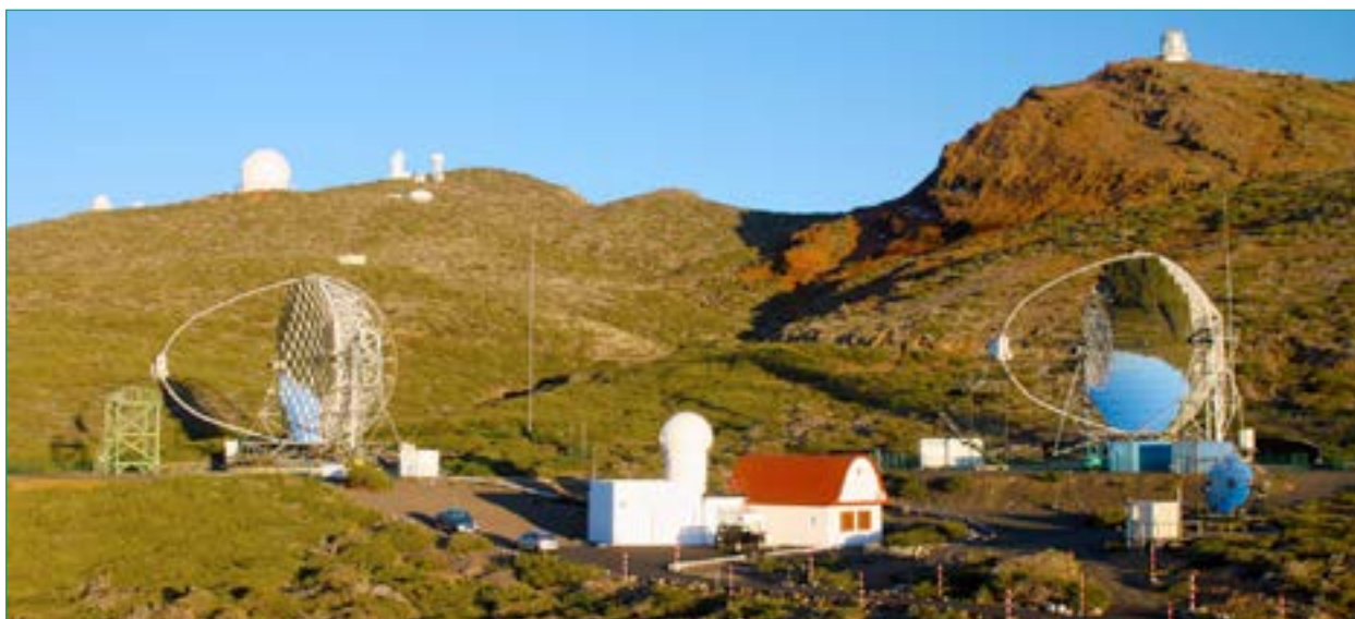
Fig. 1. The MAGIC telescopes at the Observatorio del Roque de los Muchachos in La Palma. From left to right: MAGIC-I, control house and MAGIC-II. Thanks to their large mirrors, the MAGIC telescopes working in stereoscopic mode are able to detect gamma rays of energies between ~50 GeV and ~50 TeV. They are powerful eyes to observe the most violent phenomena: the non-thermal Universe. Credit: MAGIC Collaboration.
